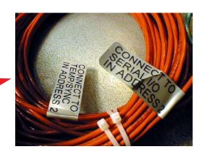
Run the Serial I/O and the TEMP/SYNC cables out of the MASTER UNIT through the communications conduit opening. Then close the sign.
